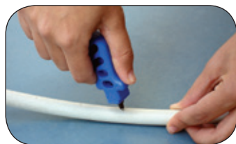
Step 1: Punch a 3mm hole in the supply line tubing.
