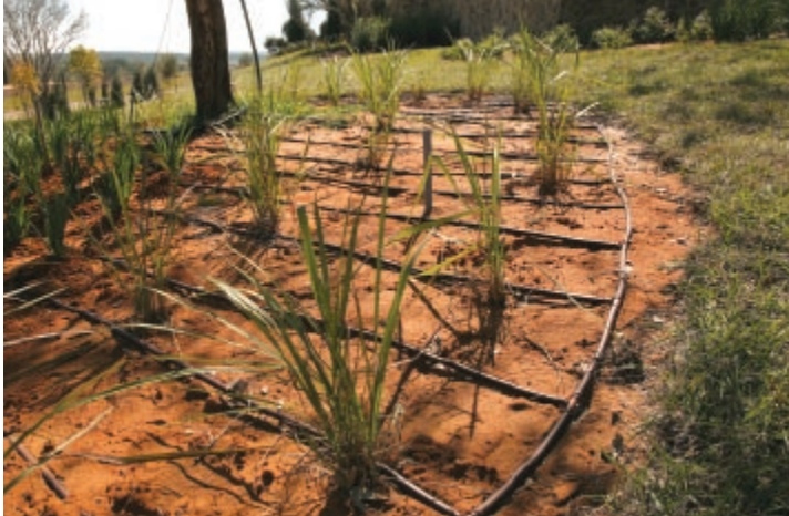
To irrigate shrub bed areas, Netafim's Techline® CV dripperline may be buried in trenches or placed on the soil surface. At Bella Collina, landscape contractor Austin Outdoor places the dripperline on the surface to help simplify installation.
