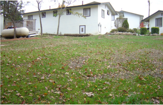
The completed drip dispersal field is now ready for use.
