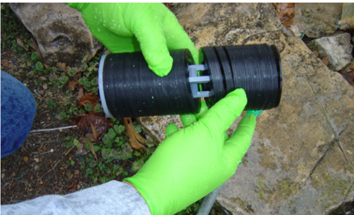
Before effluent is pumped to the drip field, it passes through a Netafim disc filter. Cleaning the discs is as easy as rinsing the rings with a garden hose. Disc filters capture over 50% more debris than screen filters by forcing the water through an overlapping grid of capture points.
