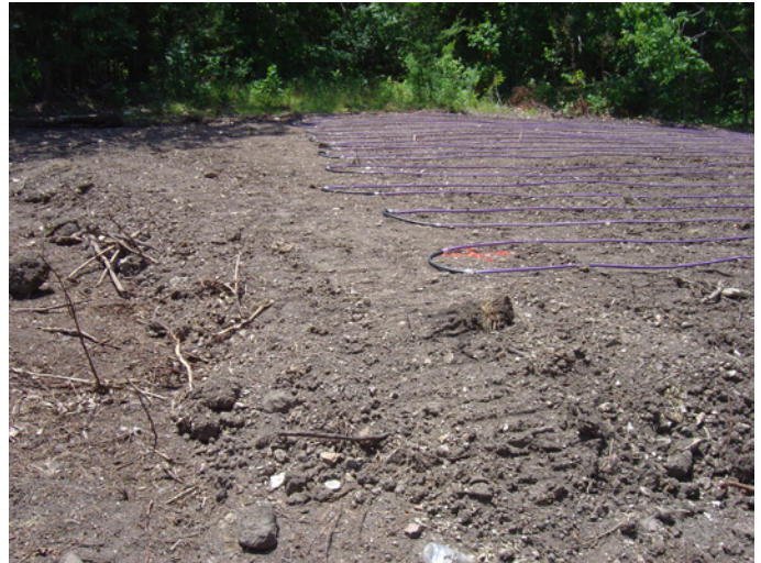
A good view of the imported base brought in for the field. Soil was brought onto the field in 4" - 6" lifts until an adequate base was established.
