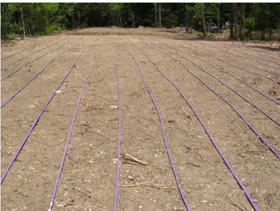
Netafim Bioline laid onto the imported soil in equally-spaced rows.
