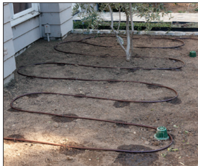
Techline dripline placed in flower beds, on top of the ground, ready to be covered with mulch.
