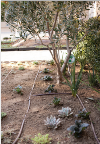
Techline dripline placed in flower beds, on top of the ground, ready to be covered with mulch.
