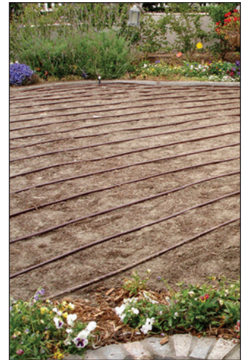
Techline dripline subsurface installation prior to laying sod.
